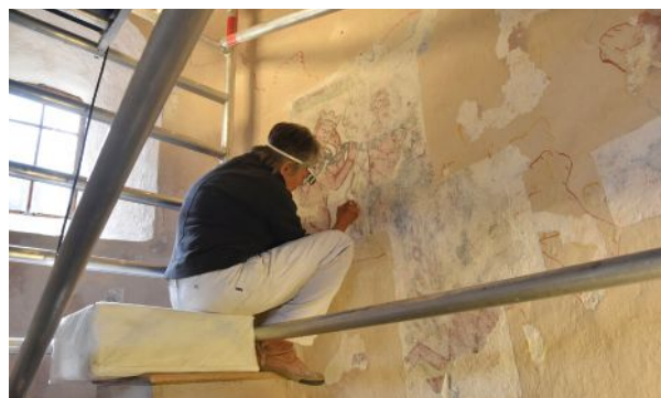
A craftsman restores a fresco at the Convent of St. John in Switzerland.
