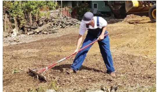
Lion Gregory Sheldon works to spread woodchips at the site.
