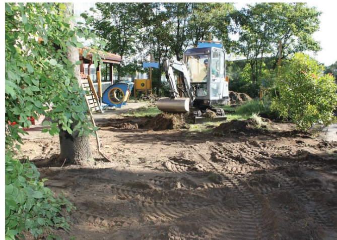
Right: The hills were evened out and weeds and pieces of concrete removed, replaced with new grass, a synthetic play surface that cushions falls, and an integrational path.
