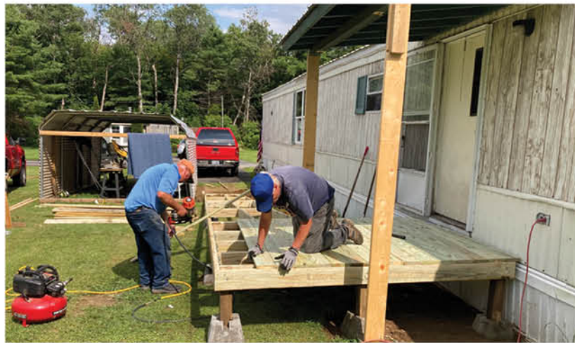
Johnstown Lions in New York built a wheelchair ramp.
